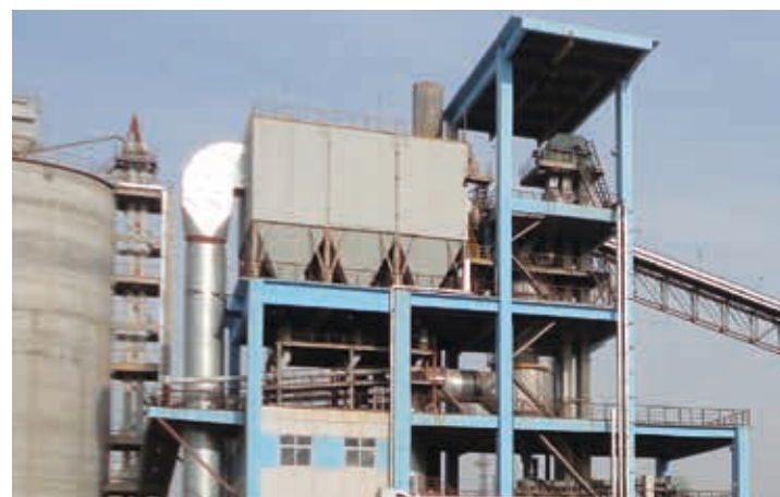
The integration of the drying function in the system.
