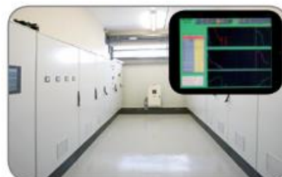
Electrical control cabinets
